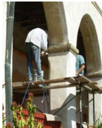
Workers replace moisture-damaged cornices in a recent project.
